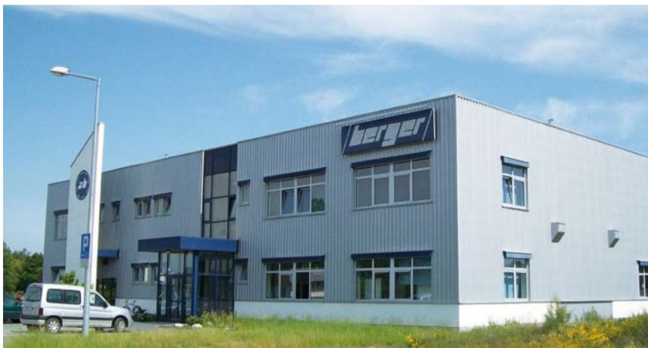
Berger plant in Kedzierzyn-Kozle, Poland.
